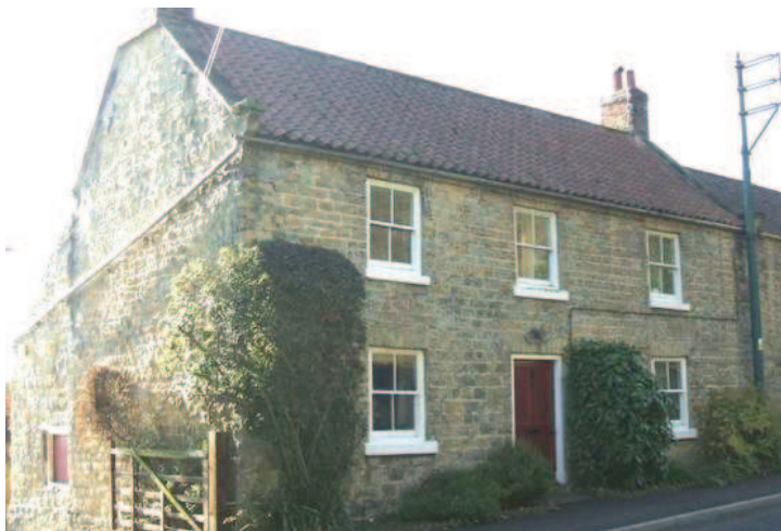
Abbey House, Main Street: coursed rubble to gable, squared stone to front
