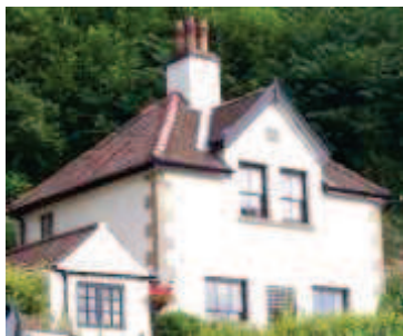
Crag Cottage, Main Street: central chimney stack
