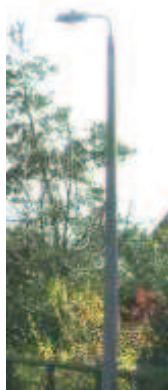
Concrete street light in Manor Close
