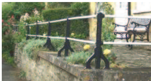
Cast iron railings along The Terrace
